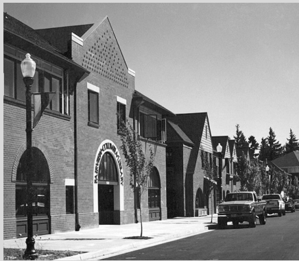
In Fairview, Oregon, the new library (above) and city hall (below) are part of a 95-acre mixed use village adjoining the “old town” neighborhood (built between 1890 and 1940). All civic buildings can be spotted by their distinctive arched entryways.
